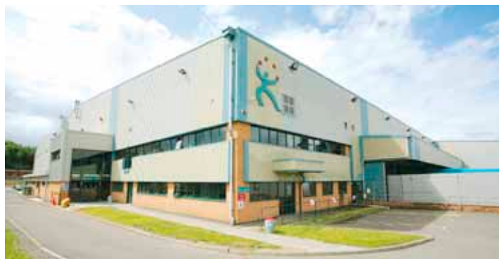
United Kingdom TDG Facility, Condor Glen, Eurocentral
