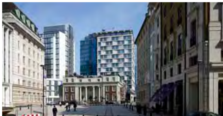
United Kingdom Premier Inn Hotel, York Road, London
