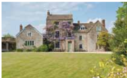
GREAT ELM, SOMERSET An impressive grade II Listed former rectory set in beautiful grounds
