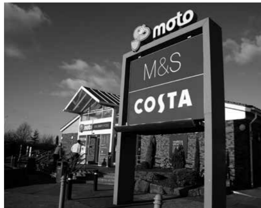
WOOLLEY EDGE MOTORWAY SERVICE AREA CLIENT: Orchard Street Investment Management ROLE: Investment valuation advice VALUE: c. £35m
